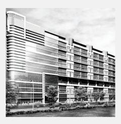
This project comprised of 8-storey multiple user clean and light industrial development. The structural system involves post tensioned flat slabs with reinforced concrete walls & cast in situ RC columns. RC flat slab is adopted for the 1st storey of the development. The structure is supported by the reinforced concrete bored piles.
