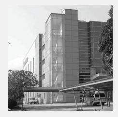
Erection of a 4-storey single user industrial development. Post tensioned beam and slab were adopted for the industrial area which are supported by the reinforced concrete columns. RC precast piles were used for the foundation.
