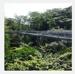
The elevated walkway of the Forest Walk is an 800 meter long walkway at an altitude of 3 meters to 18 meters above the park. The structure is built from steel and create a peaceful walk through the park.
