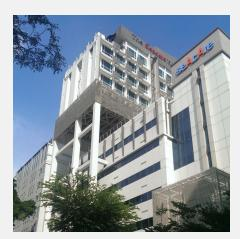
The Seacare Hotel project involved erection of a 16-storey (103 rooms) hotel block and additions and alterations works to the existing 9-storey office tower. Transfer trusses were proposed at the 13th storey to cater for the loads from the upper storey of the hotel building and support the transfer floors. All columns and beams are steel structures in order to reduce the selfweight of the building above the 13th storey.
