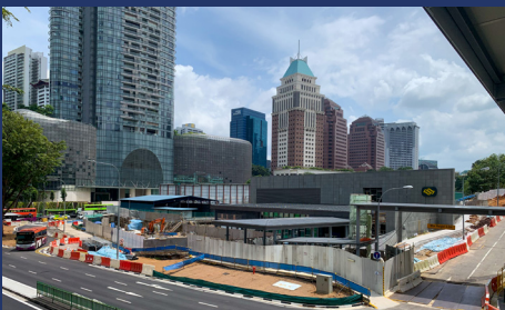
A close to completion shot of the Paterson Road exit of Orchard station (TE14).
